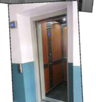
Lift at 640 Argyle Street After
