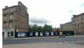
Dover St site
