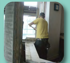
Window Replacement at 27 Derby Street
